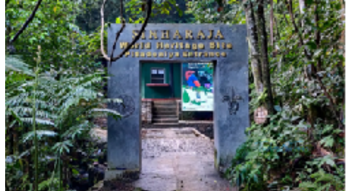
Fig. 4. The Pitadeniya Conservation and Research Centre, located in the southern boundary of Sinharaja Forest Reserve
